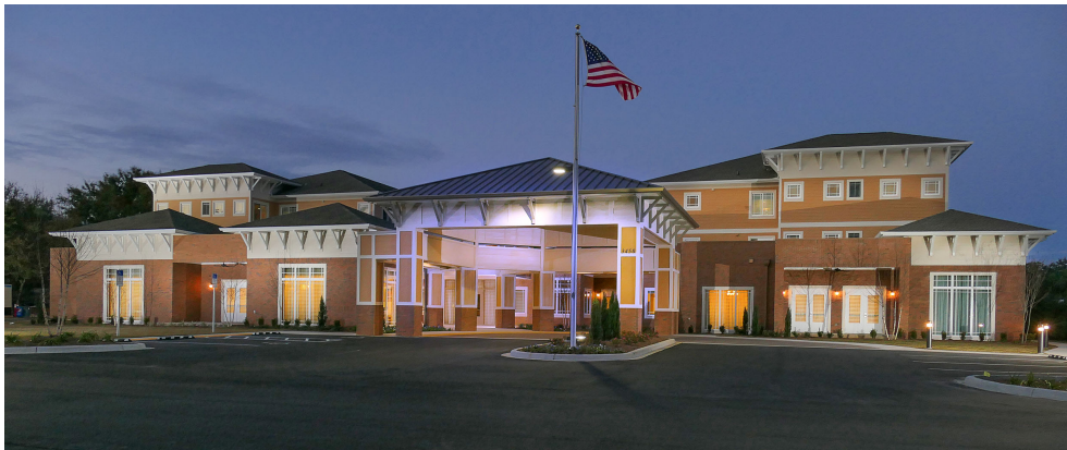
Summer Vista Assisted Living, Pensacola, Florida
